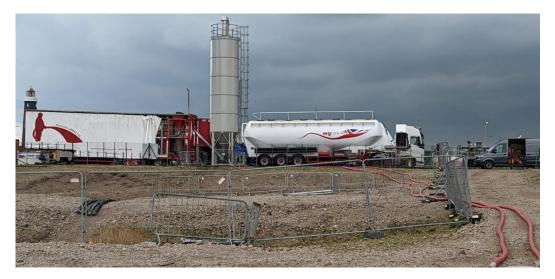
Above picture shows our batching unit set up which can manufacture 16 m<sup>3</sup> in one batch it is computerized with print off of material batched throughout the day with 1 x 38-ton vertical silo (30+ m<sup>3</sup>/hour) with 2 large grout pumps each discharging 4000 litres of grout a minute, can easily pump 500 linear meters from rear of unit.
