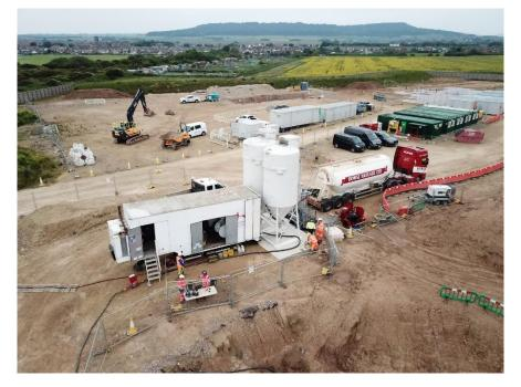
A fully computerized batching plant that can manufacture grout and light weight foam concrete with print out of tonnage used/day, 2 x 30-ton vertical silos (60+ m<sup>3</sup>/hour foam concrete, 20+ ton/hour grout) with 2 x SP 65 peristaltic pumps for discharging the material.
